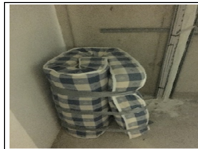
Issue ID Reference: 2.1 Example of items in the service cupboard.
